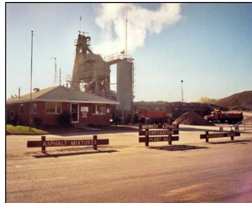
Midwest Asphalt Corporation Eden Prairie Plant
