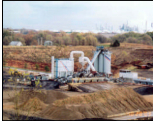
Bituminous Roadways, Inc. Inver Grove Heights and Shakopee Plants
