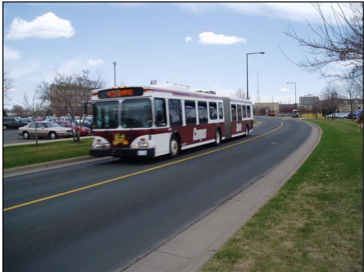
***Asphalt pavement has successfully withstood repeated heavy loads on the University of Minnesota busway between Minneapolis and St. Paul for 14 years.***
