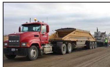
Ulland Brothers, Inc. (Albert Lea, MN) placed the asphalt pavement.
