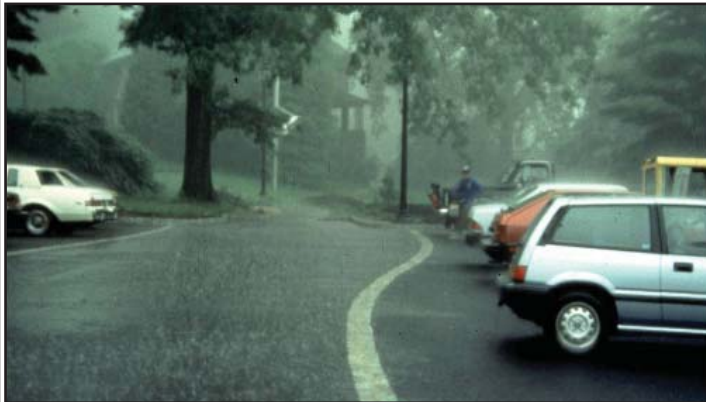
Parking lot in Pennsylvania with dense graded asphalt pavement in the driving lanes and porous asphalt pavement in the parking stalls (photo courtesy of Cahill and Associates).
