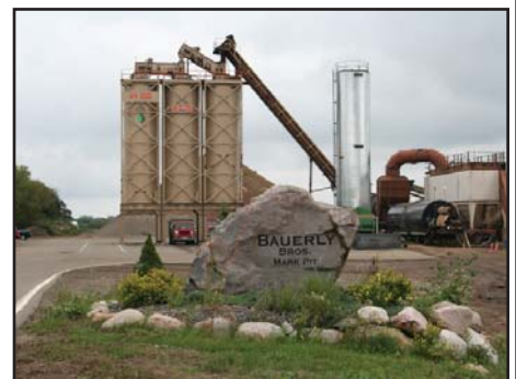
Knife River Corp. - Central MN's Plant No. 3
