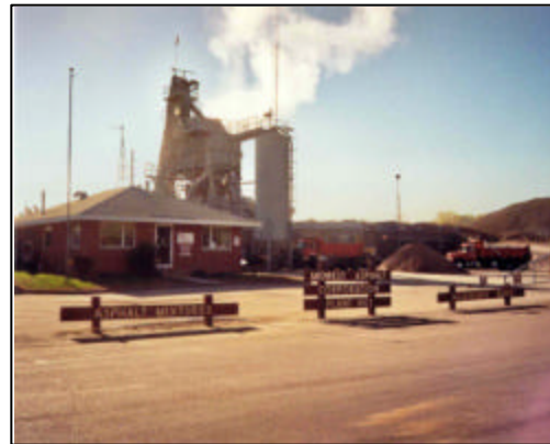
Midwest Asphalt Corporation Eden Prairie Plant
