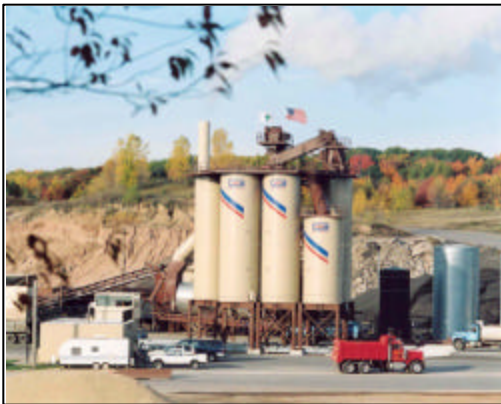
Commercial Asphalt Co. All 10 Plants (Scandia Plant shown)
