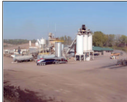
Tower Asphalt Inc. Lakeland Plant
